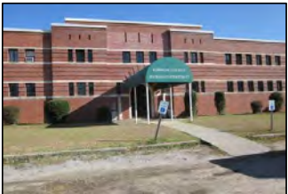
Armory Building Immediate Needs = $1,095,000
